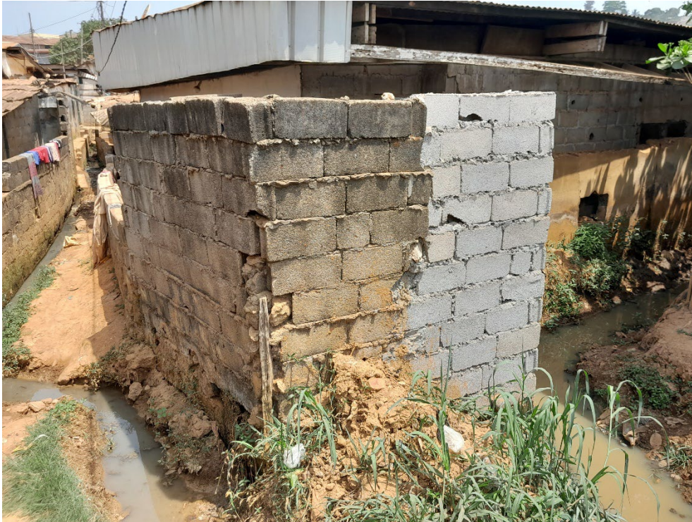
Photo 1: Toilets surrounded by waterways in an underdeveloped area in Yaounde.
