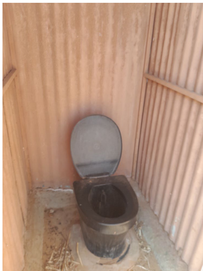
Photo 2 Toilet attached to the kindergarten. A survey on the sanitation situation in the village is one of the most important issues for the future.
